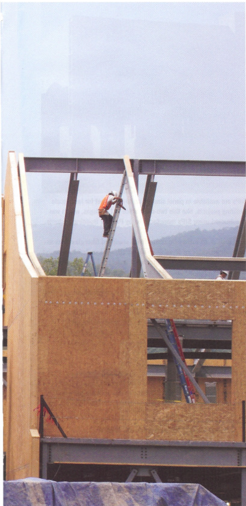
PHOTO: AL COBB, PANELWRIGHTS
