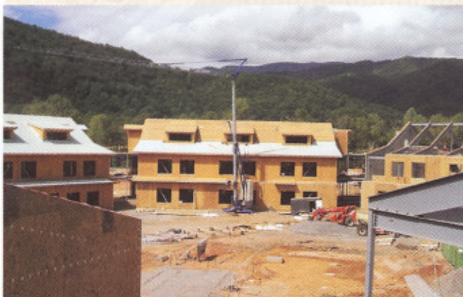
The Cherokee (N.C.) Central School is the largest project ever to be built with SIPs. In all, 376,000 sf of panels will be erected.
