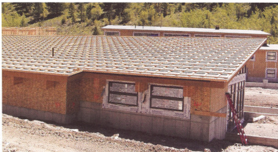
PHOTOS: PREMIER BUILDING SYSTEMS
